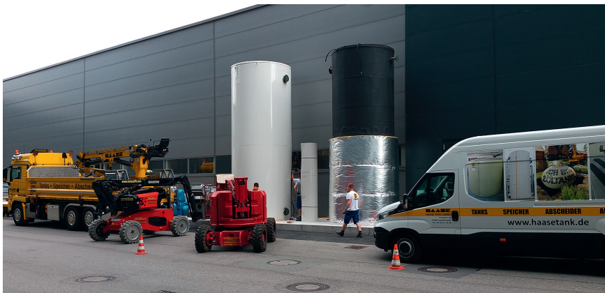
Fig. 3. Installation of insulated GFRP heat and cold storage in combination with heat pumps for heating and cooling the process water of a fruit drink producer (© Haase Tank)
